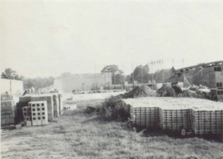
Preparation for new gym.
