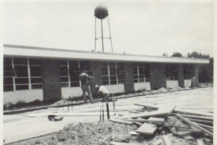
Workmen struggle to build Junior High gymnasium.
